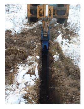
The recessed profile allows working under the pipes
